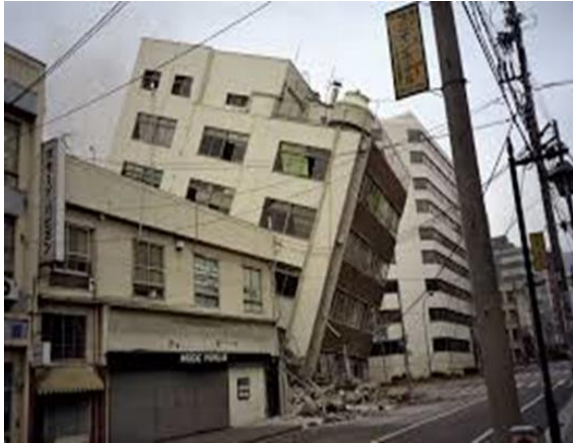
Fig.1.1. Building knocked off its foundation by the January 1995 earthquake in Kobe, Japan
